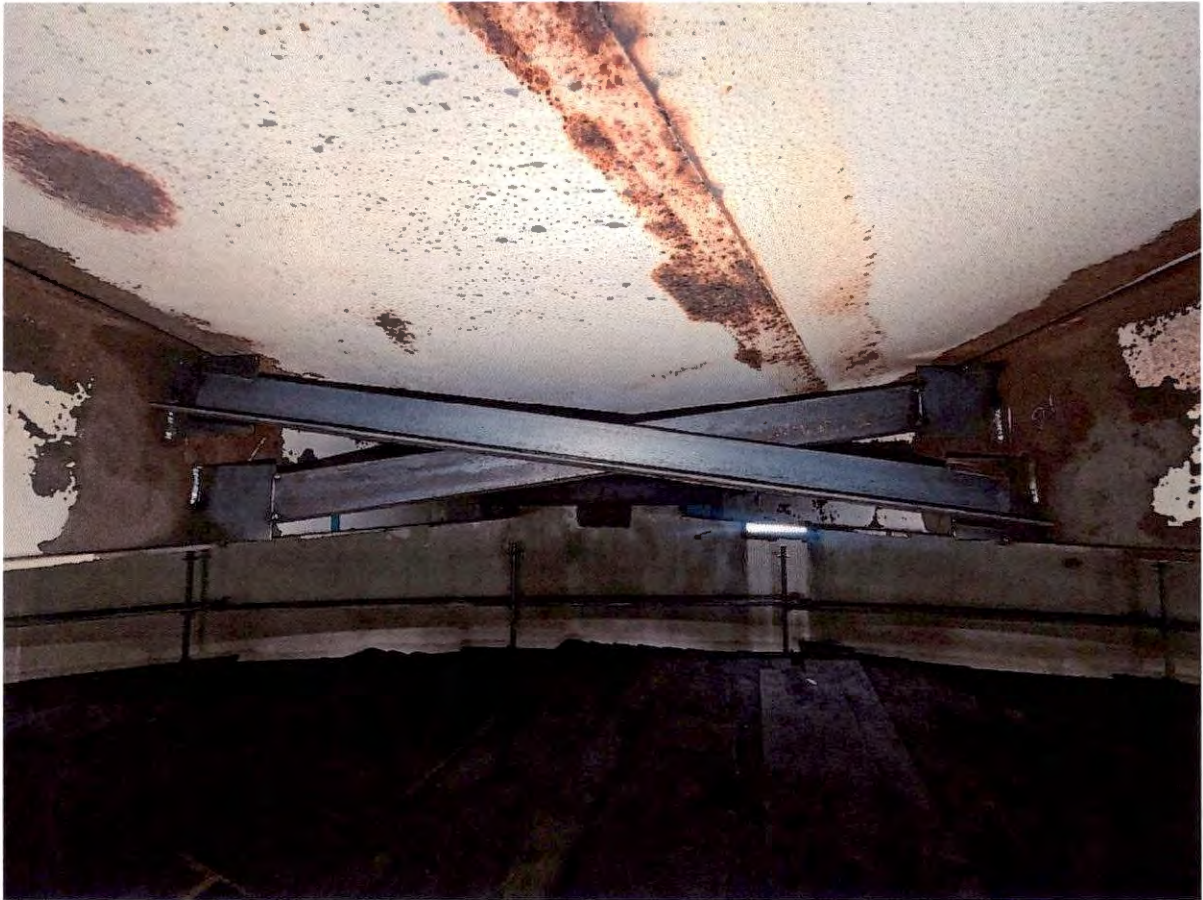
January 23, 2026 – View of rafter cross-bracing
