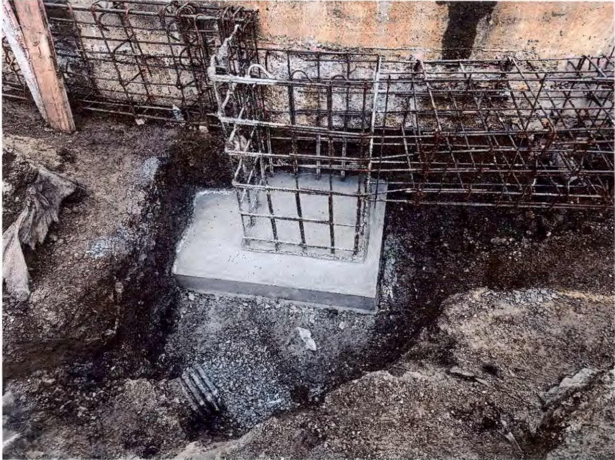
January 30, 2026 – Concrete base for the new catch basin below the overflow/drain
