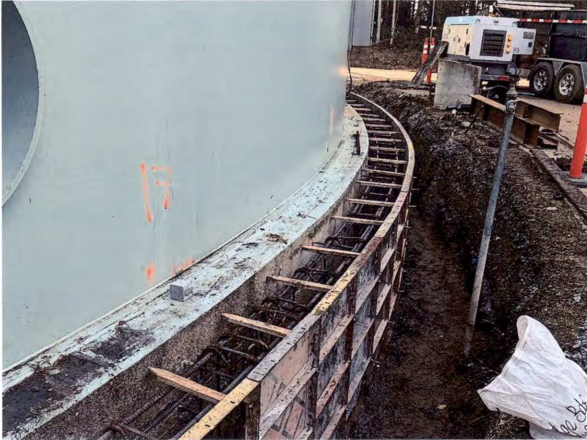
January 30, 2026 – Concrete form installation along the extended ringwall.
