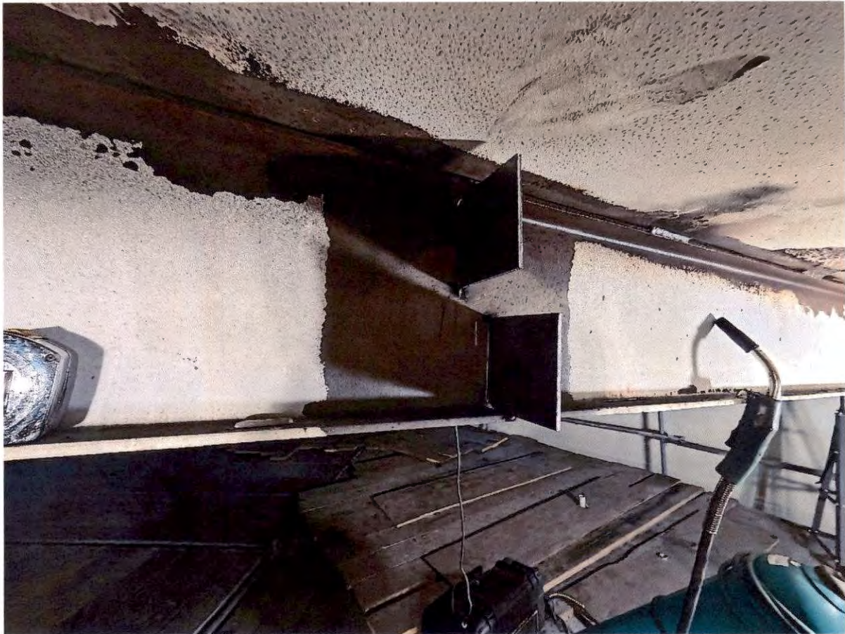
January 13, 2026 – Installation of gusset plates to permit rafter cross-bracing
